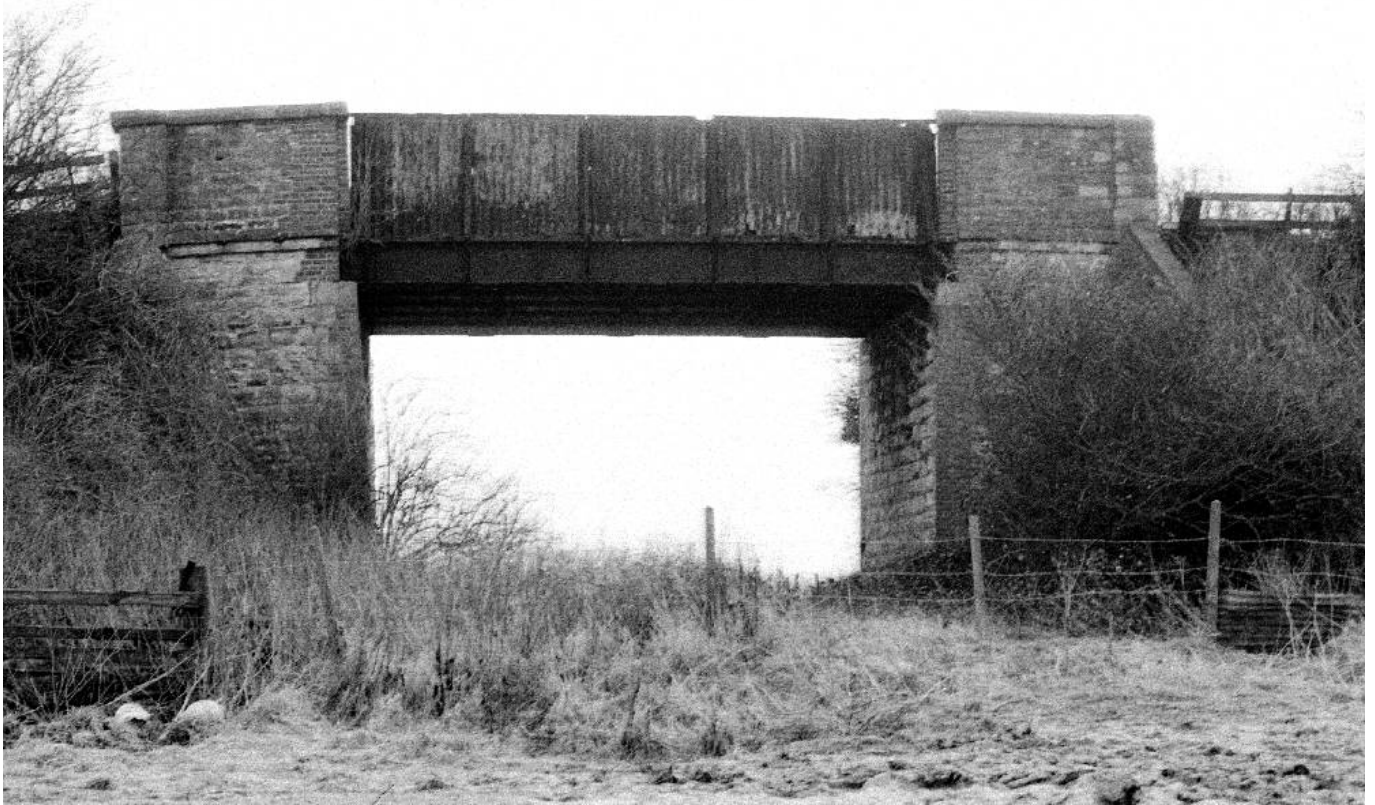
Tin Bridge before demolition
